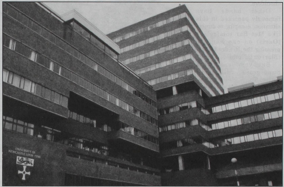
WAT-ER MESS. . . Claremont Tower where the UCS base was almost wrecked by surprise flooding
